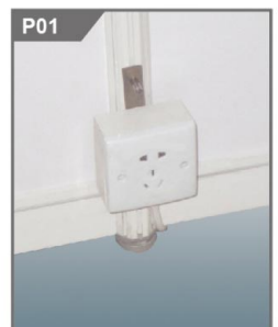
P01 插座 Power Socket (Square Pin) Max.500W
